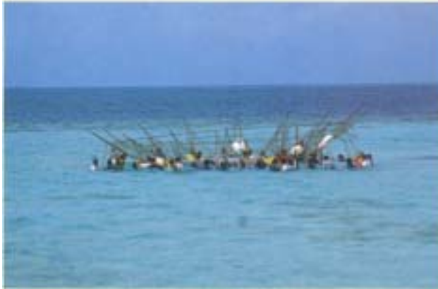
from top to bottom: Construction of the Lotus took place on the Banyan Tree beach; the Lotus was "swum" out, and released only metres from the reef's drop-off
